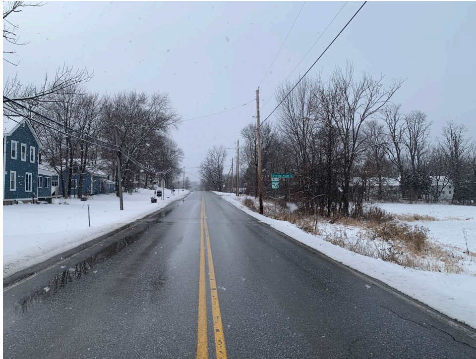
Main Street (VT Route 74) Looking East
